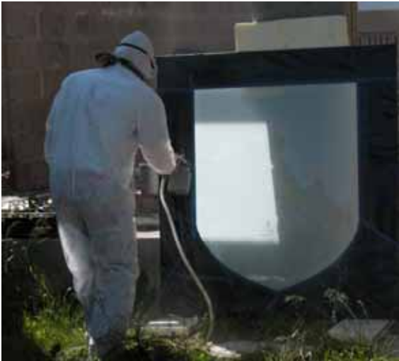
Sand blasting. Robert Emeringer.
